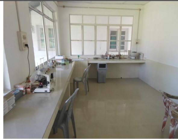
Fig 4: Construction of Laboratory.
